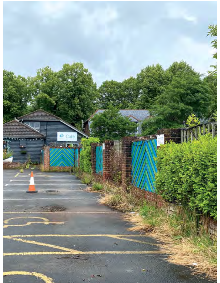
Image 6: Current impermeable parking provisions, providing little in the way of flood mitigation or retention. This is to be replaced by a variety of permeable surface treatments
